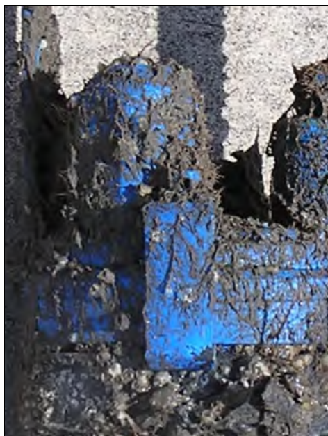
After Deployment (Close-up)
