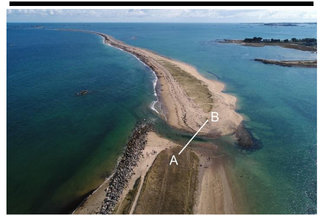
Figure 6. Breach on the sandy proximal section of the Sillon de Talbert (source: September 14, 2018). Transect A-B related to Figure 7.
